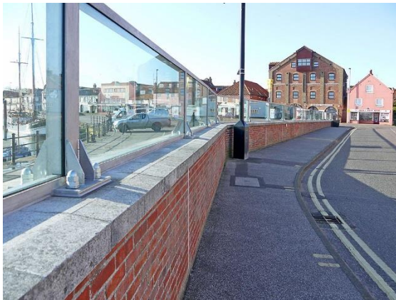
Flomsikring, foto: floodcontrolinternational.com
